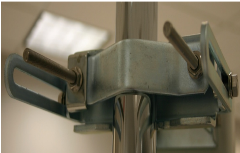
Figure 32: Attaching the AP antenna upper bracket to the pole
