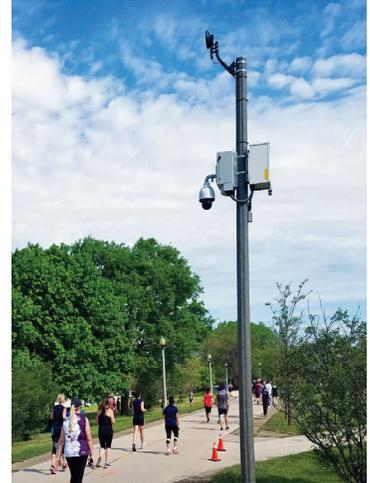
**Figure 3-1:** Pole Mount Installation
